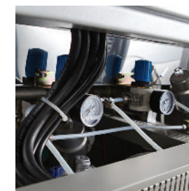
Precise Service with Descent Monitoring at Service Area
