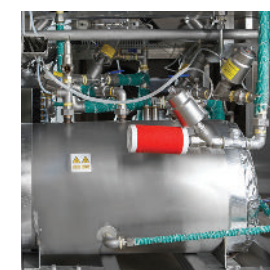
Steam Generator Made of AISI 316 L Stainless Steel
